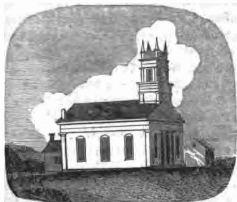
St. Stephen's Church, North Castle.
